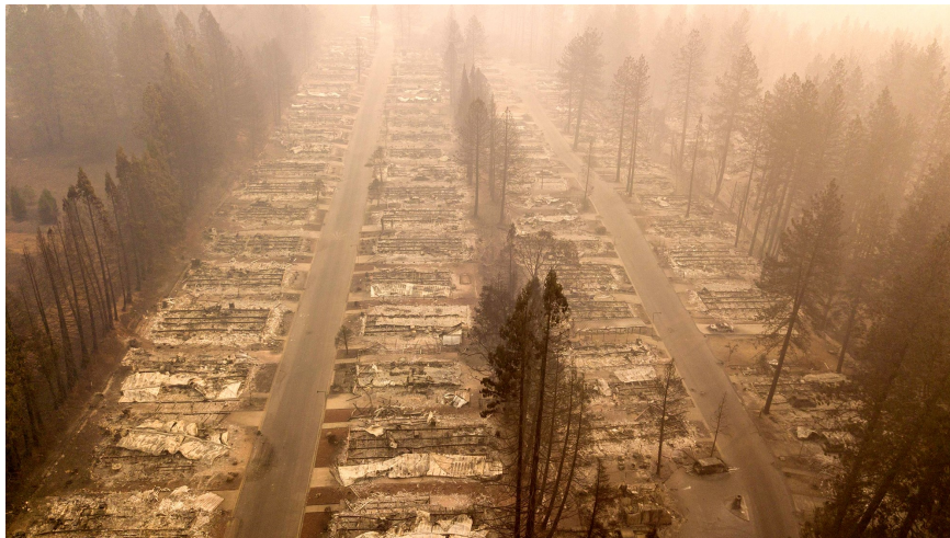
The charred remains of a neighborhood in Paradise, CA after the Camp Fire of November 2018. (Photo by Josh Edelson/ AFP - Getty Images File. Source: NBC News ( LINK ), accessed Fall 2019)
